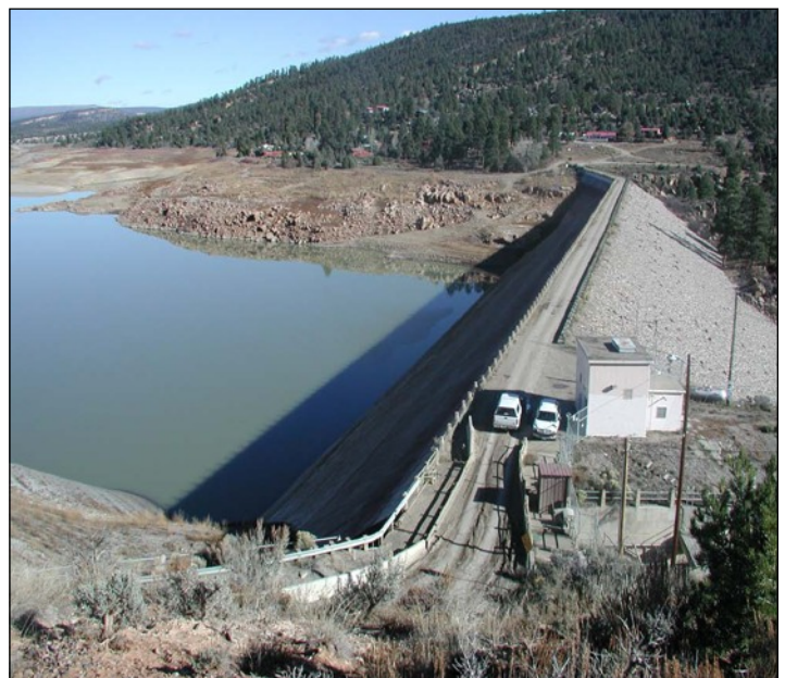
Photo Courtesy of Bureau of Reclamation Scenarios developed by Project modelers will suggest changes to operations at El Vado Dam (above).
